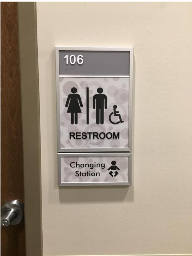
ADA-compliant interior signage that meets VA standards. Submit prototype to medical center for approval. Provide changing stations in common bathrooms in both sex bathrooms with signage.
