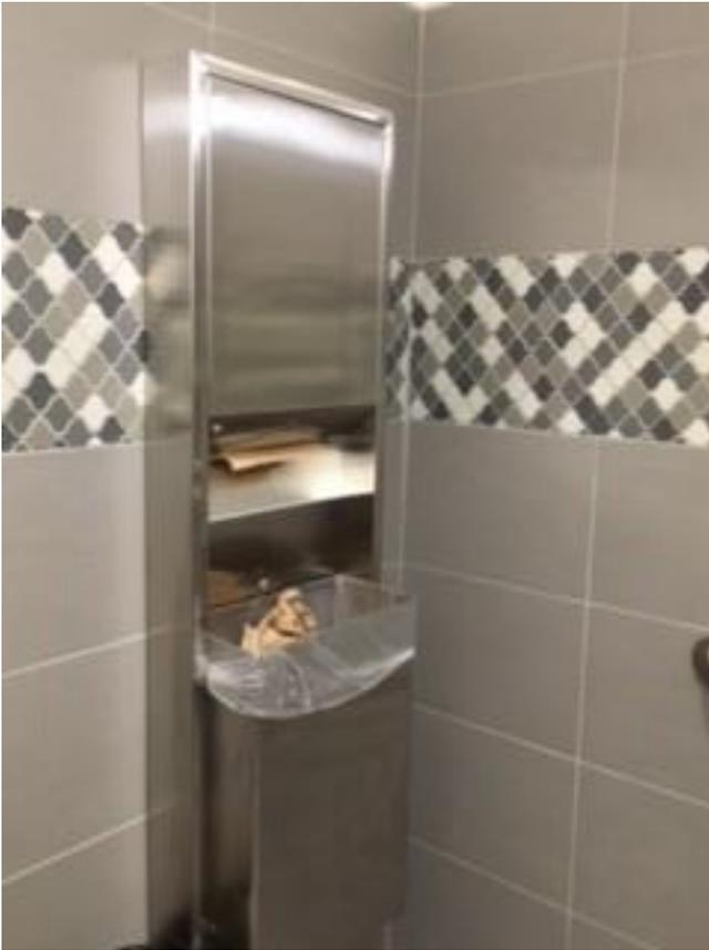
Appropriate quality materials include stainless steel, through body porcelain tile, integrated cove base and urethane grout. Interior design will assist with selections of materials and approve before purchasing.
