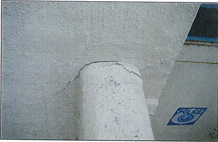
Photograph 37: Concrete Crack At Exterior Retaining Wall and North Building Face
