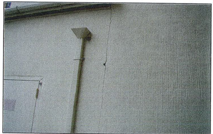
Photograph 40: Concrete Crack At North Face Exterior Wall
