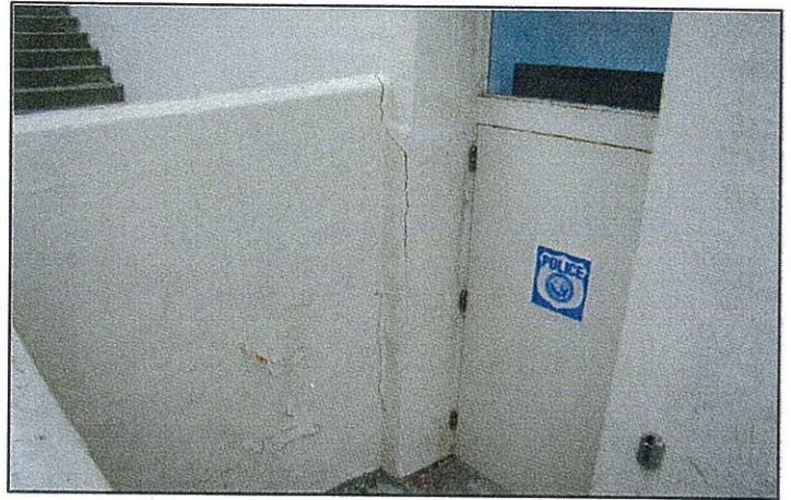
Photograph 38: Concrete Crack At Exterior Retaining Wall and North Building Face
