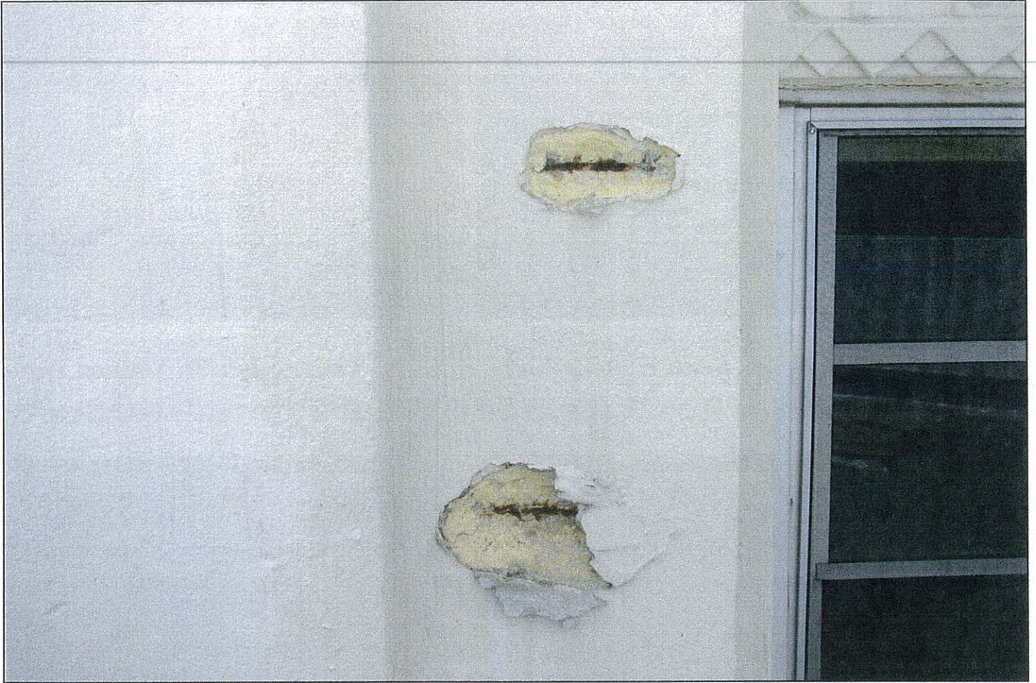
Photograph 47: Failed Spall Repairs
