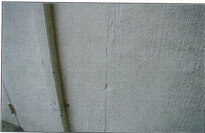
Photograph 39: Concrete Crack At North Face Exterior Wall
