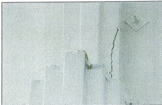
Photograph 44: Concrete Spall
