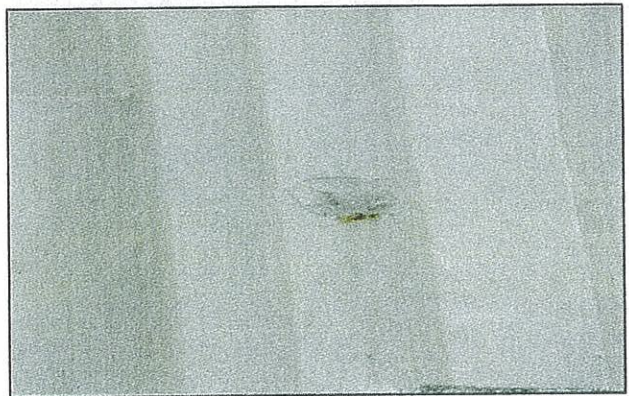
Photograph 43: Typical Concrete Spall with Corroded Reinforcing
