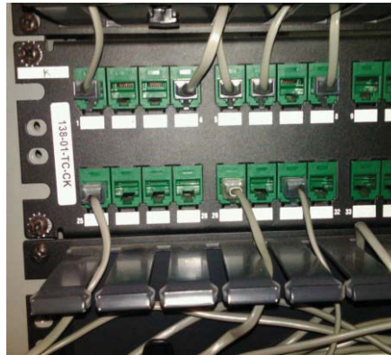
Figure 4: Wall Phone patch panel
