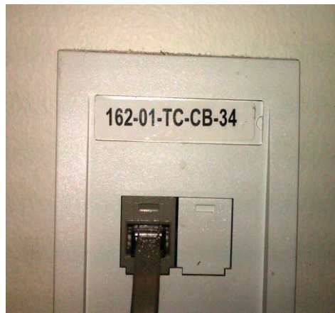
Figure 1: Faceplate showing labeling scheme.
