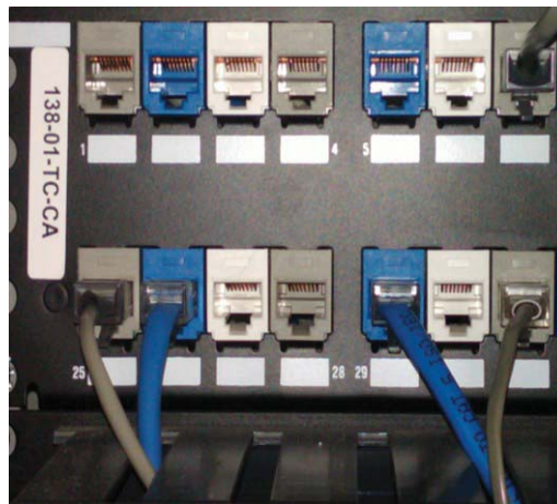
Figure 3: Patch Panel Example
