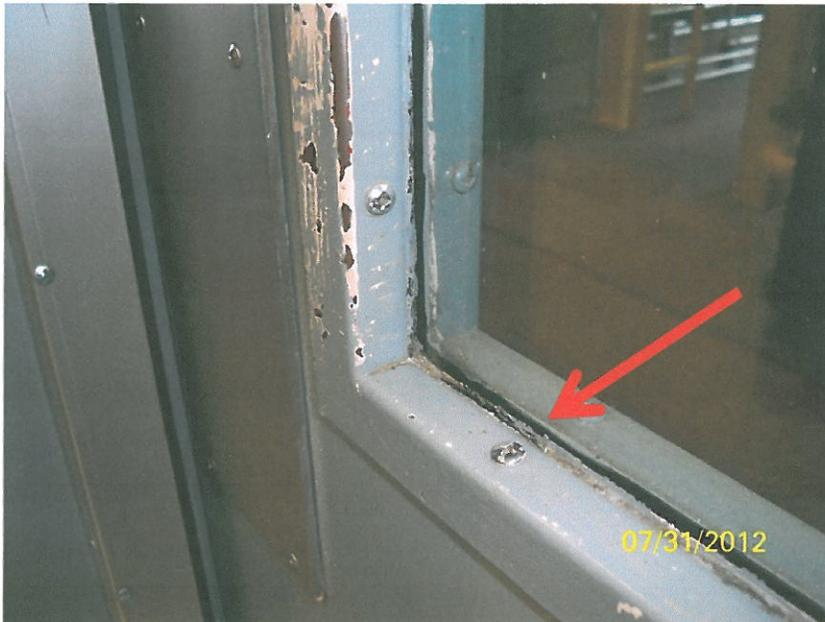
**NO SUSPECT ACM WAS IDENTIFIED PRESENT ON THE BURNER ITSELF OR ON THE EQUIPEMENT TO BE DISTURBED ASSOCIATED WITH BOILER #3. THE WINDOW GLAZING ON THE CONTROL ROOM DOORS WAS THE ONLY SUSPECT MATERIAL SAMPLED IDENTIFIED TO BE ASBESTOS CONTAINING BY THE LABORATORY. NO LEAD BASED PAINT WAS IDENTIFIED IN ANY OF THE AREAS OR ANY EQUIPMENT DETERMINED TO BE DISTURBED.**
