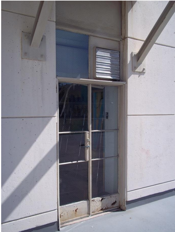
14. Corroded Steel Patio Doors near Chapel
