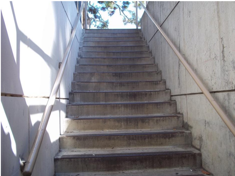
13. Non- compliant handrail at basement stairs
