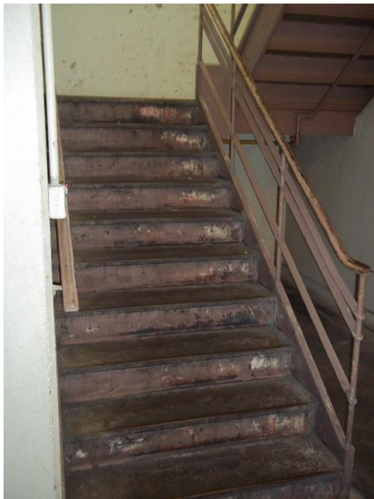
10. Damaged, non-compliant handrail @ basement stair to Canteen
