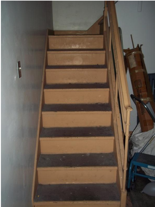
5. Non-compliant Mezzanine Stair
