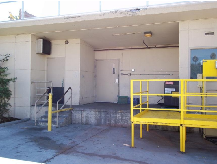
4. Non-Compliant Handrail
