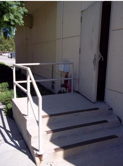
3. Corroded Hand-rail
