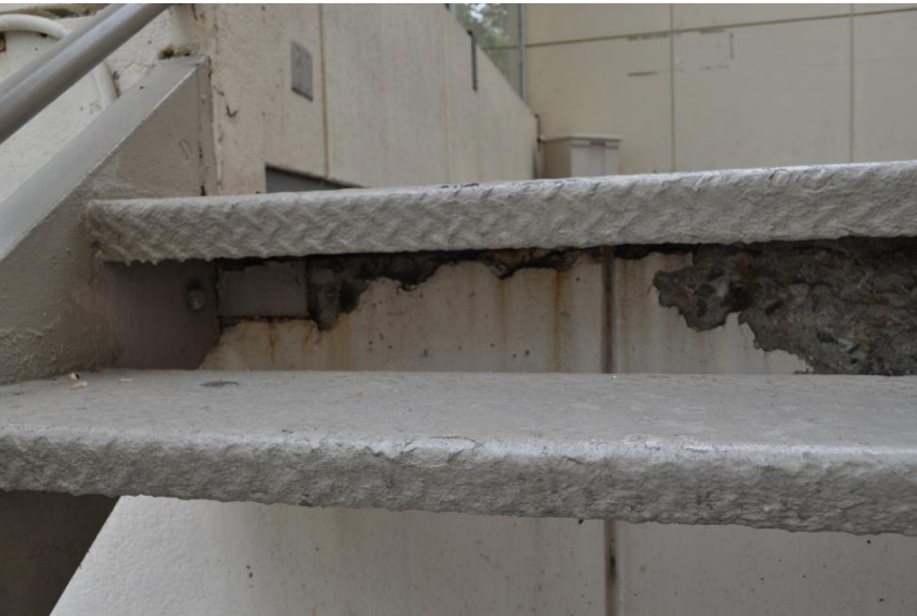
2. Spalling at Exterior Stair
