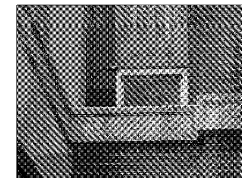
ELECTRIC CONDUIT THROUGH WINDOW JAMB
