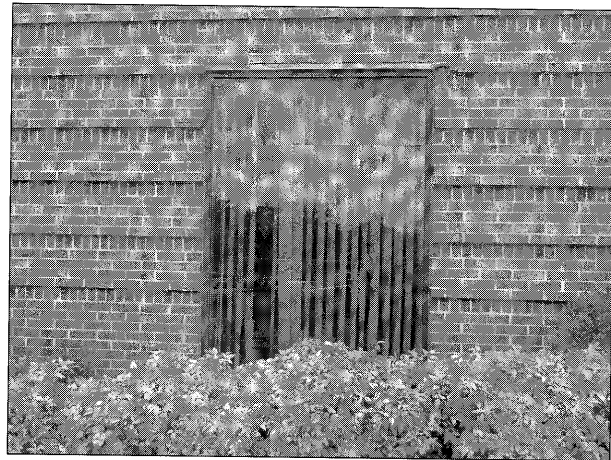
REPLACE 3 COURSE OF BRICK & REPLACE WINDOW LOCATED ON C-WING. SEE CALLOUTS 1 & 2
