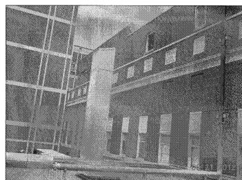
REPLACE THE TWO PENTHOUSE WINDOWS LEVEL THREE WINDOWS ARE COVERED IN BRICK VIEW OF WEST SIDE OF C-WING SEE CONSTRUCTION NOTES A, B, & C.
