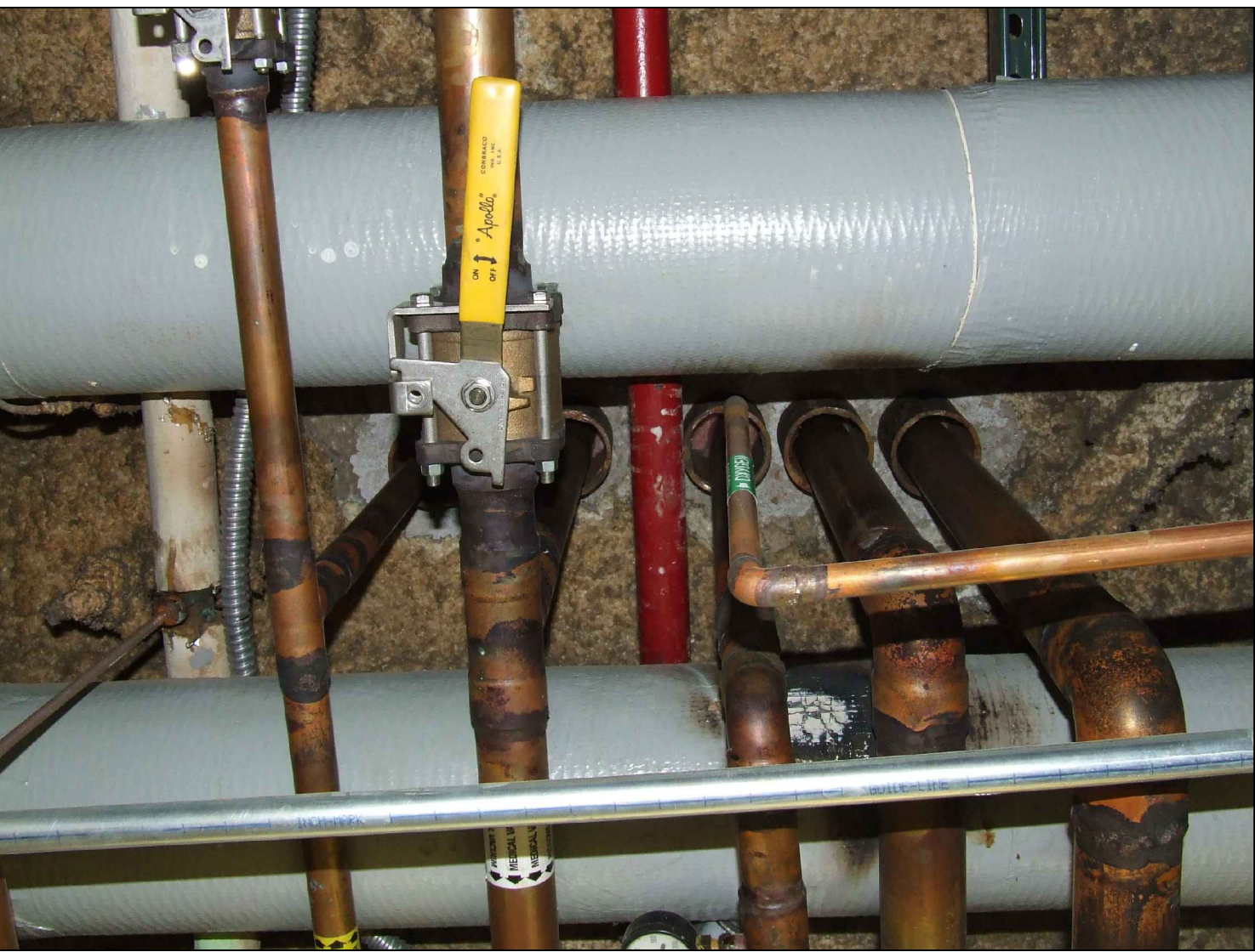
PHOTO TAKEN IN GROUND FLOOR OF MEDICAL GAS PENETRATION THROUGH FIRST FLOOR CONTRACTOR TO WORK AROUND MEDICAL GAS WHILE RENOVATING FIRST FLOOR. FLOOR PLAN MAY BE MODIFIED AS NOT TO DISTURB MEDICAL GAS SYSTEM
