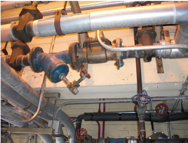
Multiple steam lines, valves and elbows lacking proper insulation.
