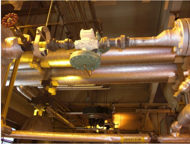
Insulation missing on valves
