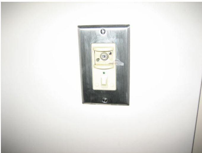
Sensor plant broken
