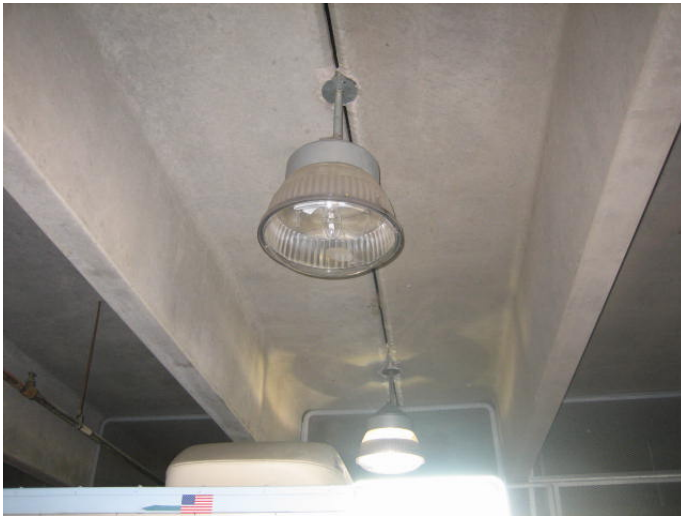
Photo 5 parking garage typical MH mounting arrangement
