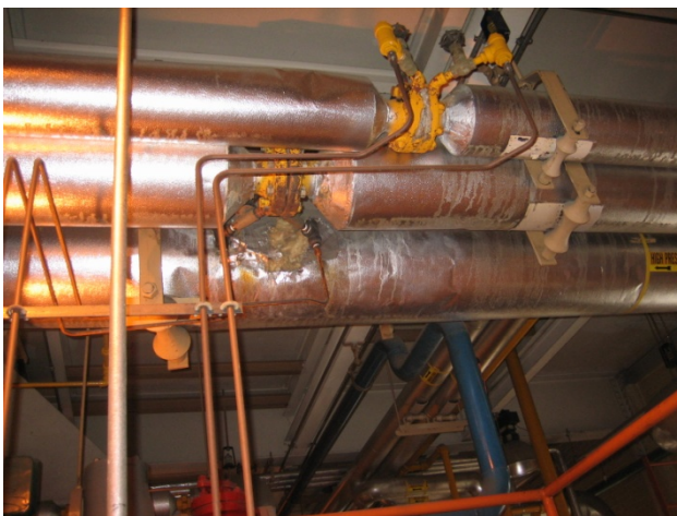
Missing insulation on valves in Boiler room
