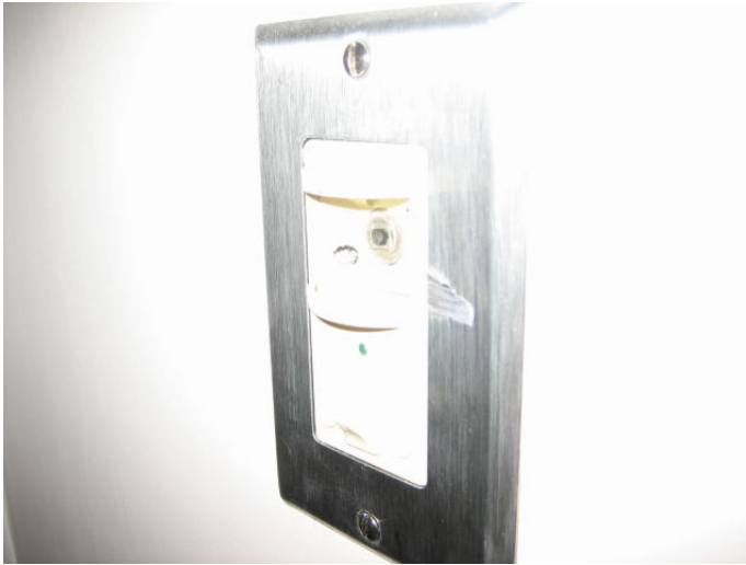
Broken and damaged sensor
