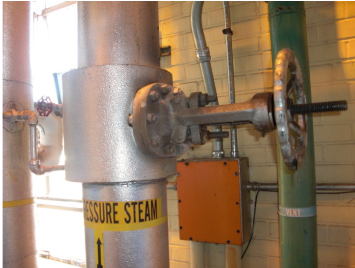
High Pressure Steam shut off Valve several
