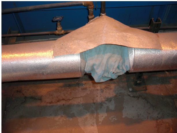
Damaged insulation/blanket at piping intersection
