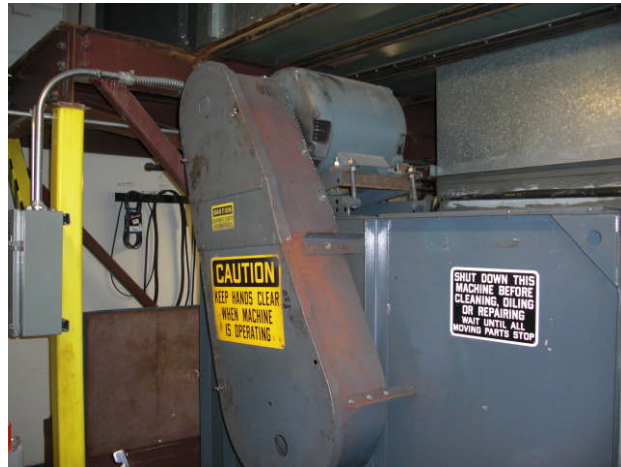
Figure 6 - Supply fan 5
