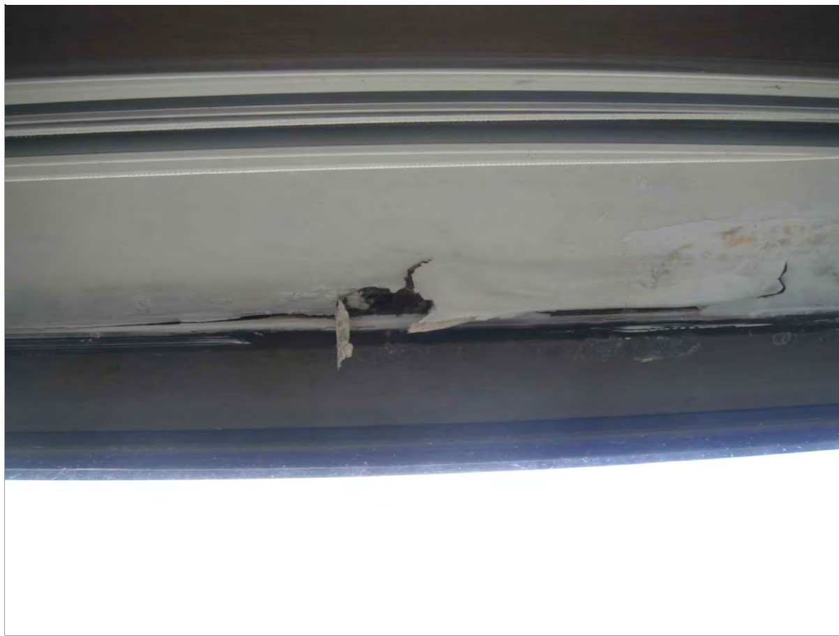
REPAIR INTERIOR WINDOW HEADER THAT HAS WATER DAMAGE LOCATED IN THE WAITING ROOM
