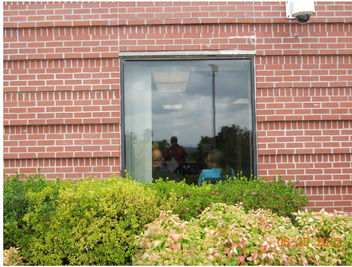
REMOVE 3 COURSES OF BRICK & REPLACE WINDOW LOCATED ON C-WING. SEE DETAL 2/A1.5
