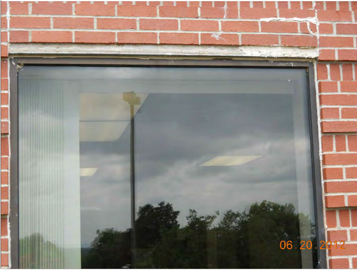
REMOVE 3 COURSES OF BRICK & REPLACE WINDOW LOCATED ON C-WING. SEE DETAIL 2/A1.5
