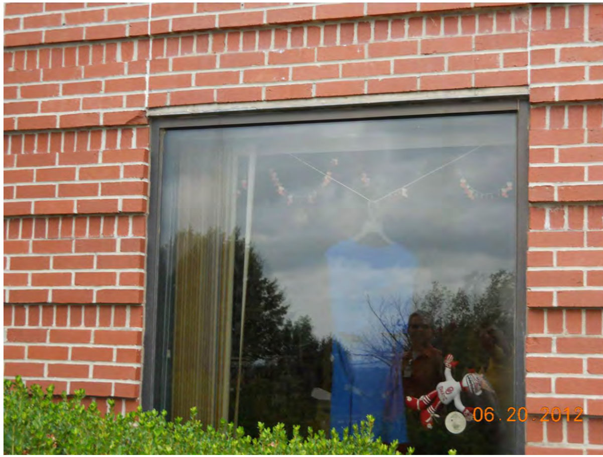
REMOVE 3 COURSES OF BRICK & REPLACE WINDOW LOCATED ON C-WING. SEE DETAILS 2/A1.5
