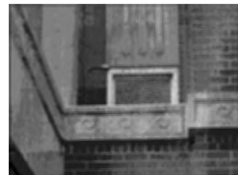
ELECTRIC CONDUIT THROUGH WINDOW JAMB
