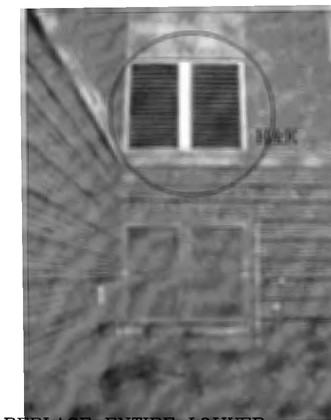
REPLACE ENTIRE LOUVER SEE CONSTRUCTION NOTES H LOCATED BY CHAPEL SOUTH B-WING
