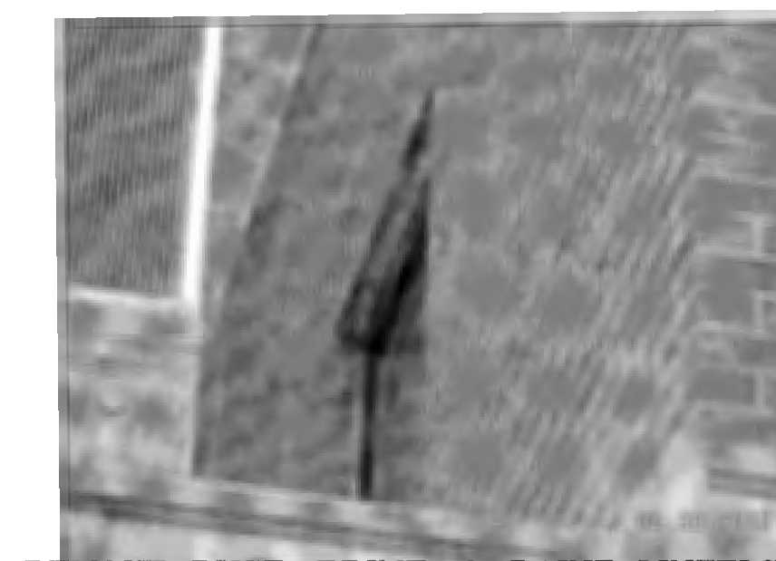
REMOVE RUST, PRIME, & PAINT LINTELS LOCATED BY CHAPEL SOUTH B-WING
