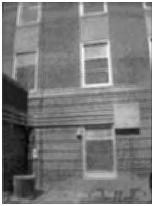
ELECTRIC CONDUITS LAY ACROSS WINDOW HINDERS THE CONSTRUCTION PROCESS ALSO REMOVE RUST, PRIME, & PAINT DOOR SEE CONSTRUCTION NOTE M.
