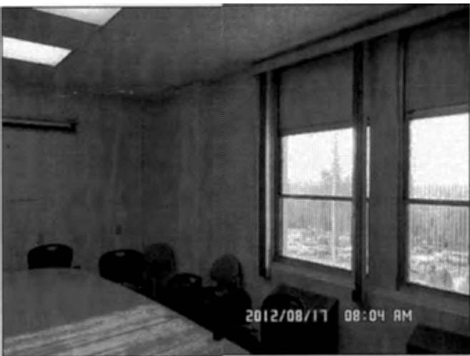
SHOWS HOW THE CEILING OVERLAPS WINDOWS REPLACE VERTICAL BLINDS LOCATED IN THE CONFERENCE RM
