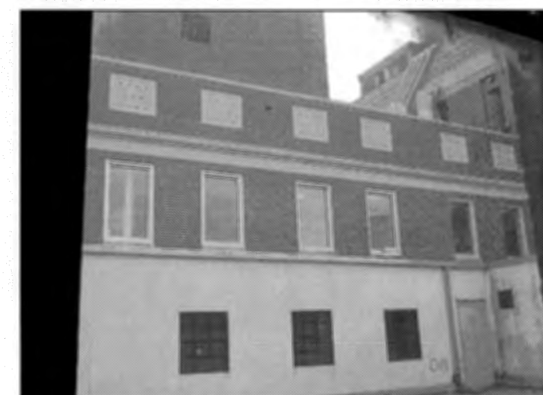
REPLACE THREE .90 LAMINATED WINDOWS WITH AN 8" O.C. GRID BETWEEN GLASS LOCATED ON C-WING WEST ELEVATION
