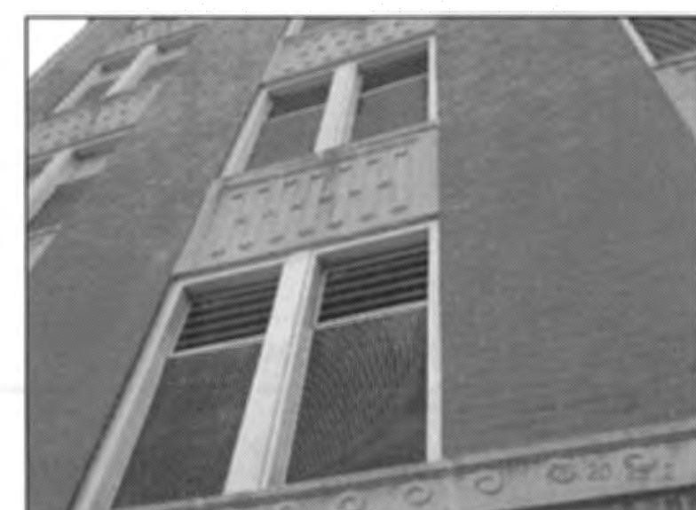
REPLACE LOUVER & WINDOW COMBINATION LOCATED ON A-WING NORTH ELEVATION
