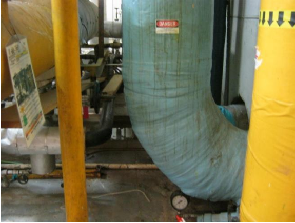
1. Sample Area #1 Pipe Mastic – 5% Chrysotile
