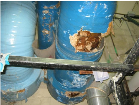
5. Sample Area #5 Pipe Mastic – 5% Chrysotile
