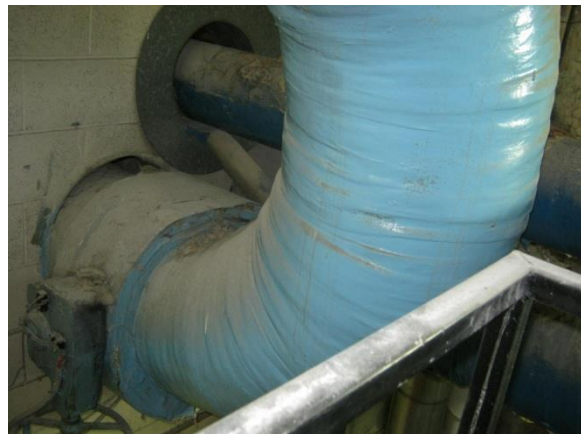
6. Sample Area #6 Pipe Mastic – 5% Chrysotile
