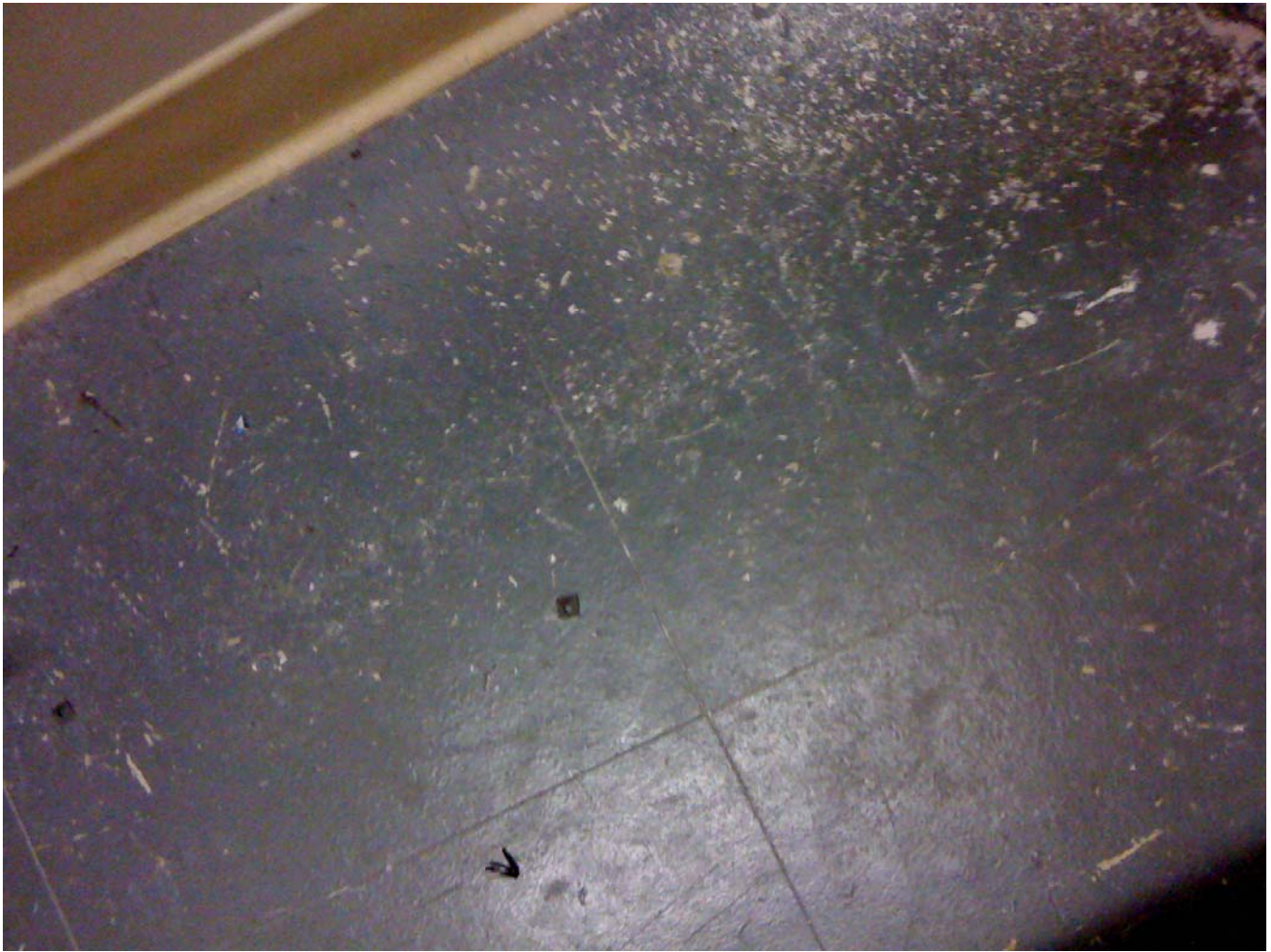
Building 23 Sample 37 Tile - 12" x 12" Grey Floor Tile and Mastic
